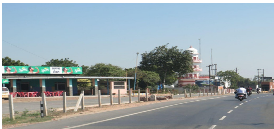
Picture showing absence of guard rails
