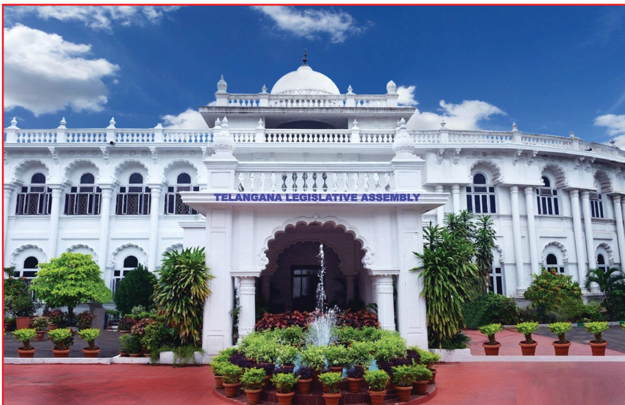
Telangana Legislative Assembly Building
